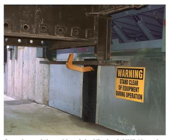
Once the truck is positioned the Ultrahook UHR40 reaches out and pulls in to hook and securely hold the trailer while loading / unloading takes place. The only component that extends beyond the pit is the heavy-duty steel hook.
